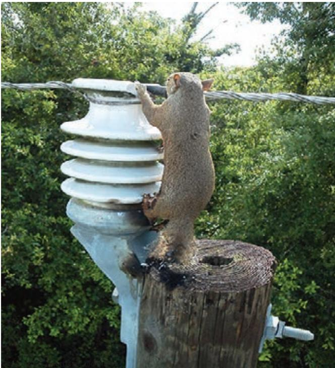
CECA makes every effort to protect wildlife from encountering harm on our lines and equipment. In addition to design specs that minimize damage, we also use insulated bird wire and insulated bushing. However, birds, squirrels, snakes and even ants, as well as livestock can cause blinks.
