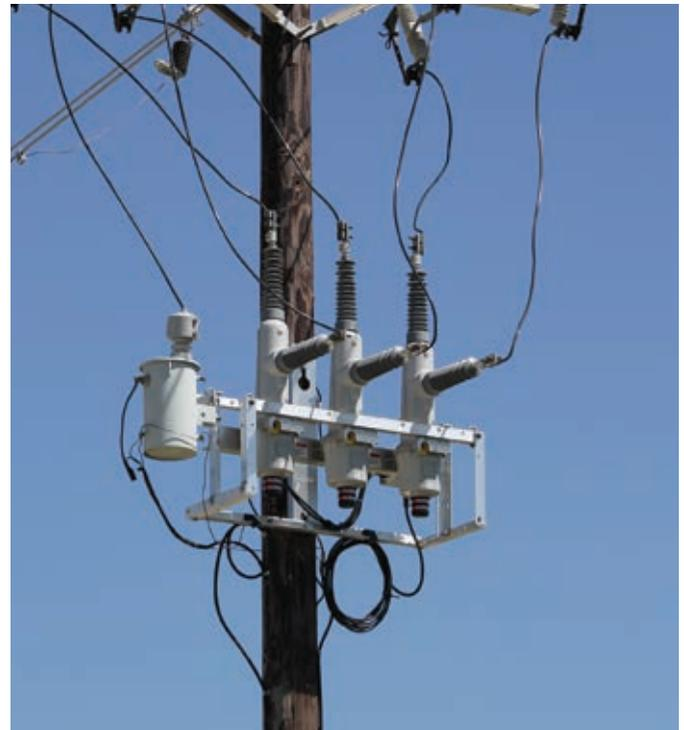
In electric power distribution, oil circuit reclosers are used on overhead distribution systems to detect and interrupt momentary faults. Because many short circuits clear themselves, a recloser improves service continuity by automatically restoring power to the line after a momentary fault.
